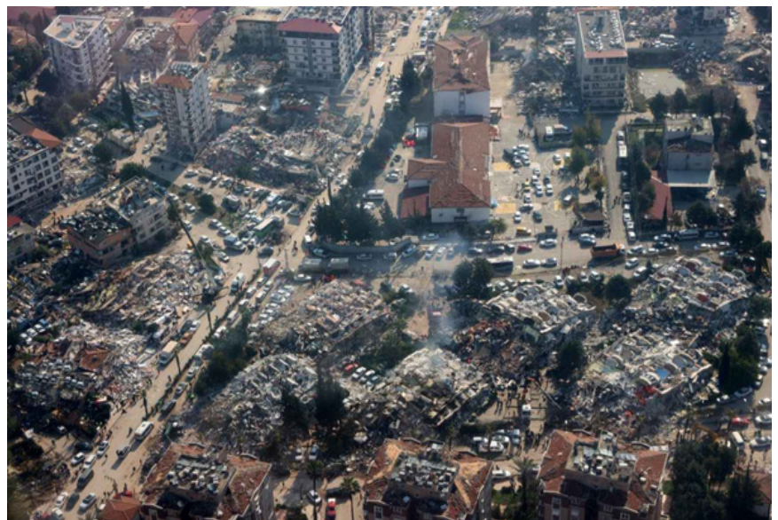
Figure 1: Kahramanmaraş earthquake in Turkey
